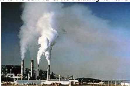
*Pic: Before fuel gas desulfurization was installed, the air-polluting emission from this power plant in New Mexico contained excessive amount of sulfur dioxide (Wikipedia)*
